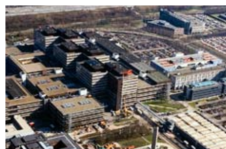
AMC Hospital, Nederländerna Hospital Solution
